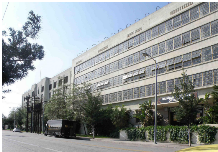
Figure 1) Exterior of Lincoln Heights Jail
