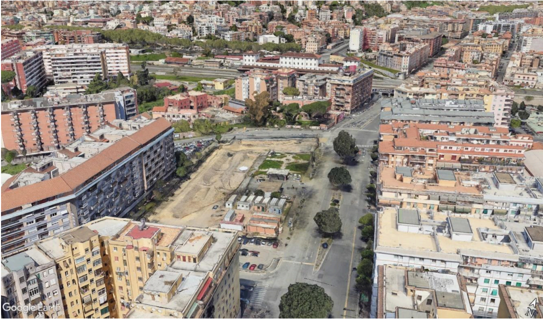
Figure 2 - Piazzale della Radio. Above left the incomplete areas towards the railway embankment. Source: Google Earth
