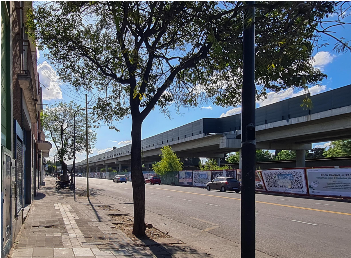
Figure 8) The train has been recently elevated, but the urban barrier persists. Ph: María Emilia Persico.
