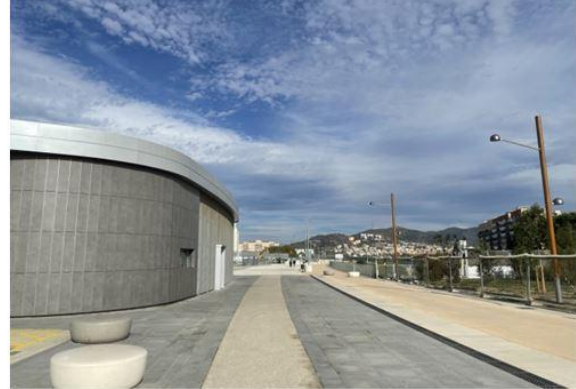
Figure 7: New pedestrian platform above the rails.
