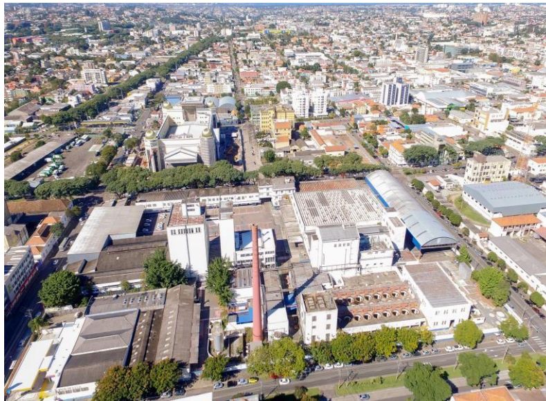
Figure 1: Aerial view of the Vale do Pinhao area (Source: IPPUC/PMC)
