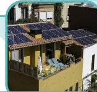
Solar Panel Installation/Retrofitting
