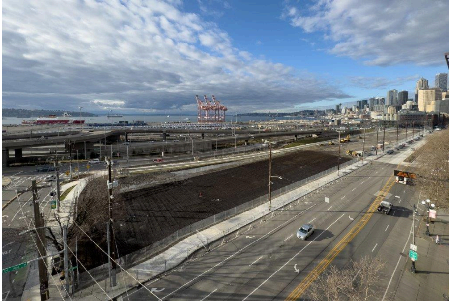
Figure 2: The WOSCA site in February, 2024 looking in a northwest direction. The site includes all of the vacant land in the image including the land stretching towards the buildings in the photo. First Ave. S. is in the foreground.
