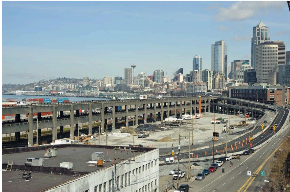
Figure 4: The WOSCA site in April, 2011 looking in a northwest direction, before the State Route 99 viaduct was removed. The viaduct is now replaced with an underground tunnel, which made possible an extensive program of waterfront open space and public realm improvements along Seattle's central waterfront. The warehouse structure in the foreground and viaduct ramps seen in this photo have also been removed.
