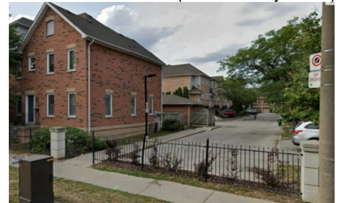
Thorncliffe Townhouses (Adjacent to Project Area)
